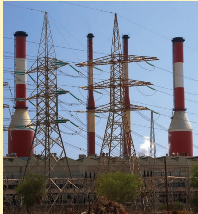
Oil-fired power station in Cyprus – indirect costs are a very high proportion of total costs in electricity generation
