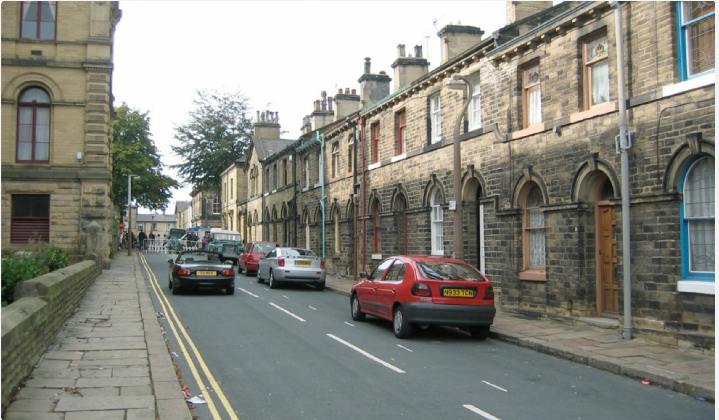
Workers' Housing - fronts
