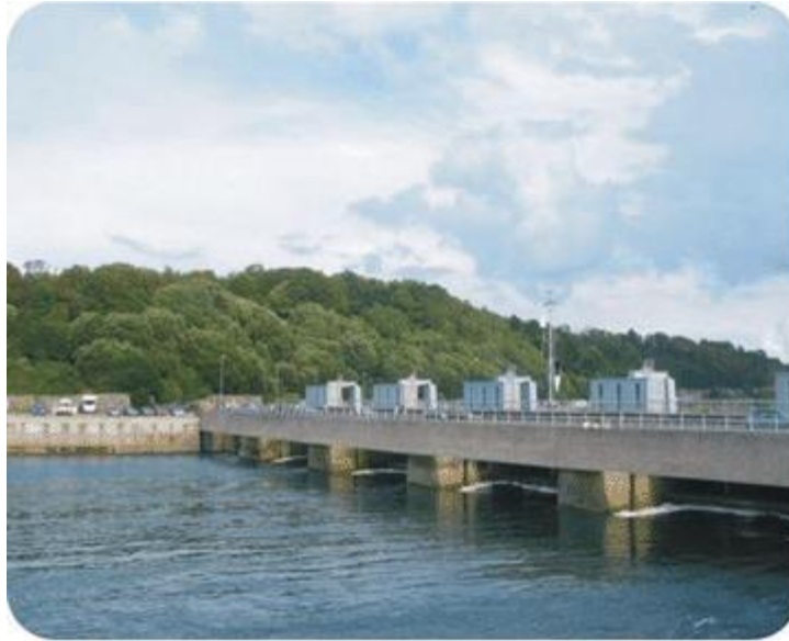
Dam of the tidal power plant in the Rance River, Bretagne, France
